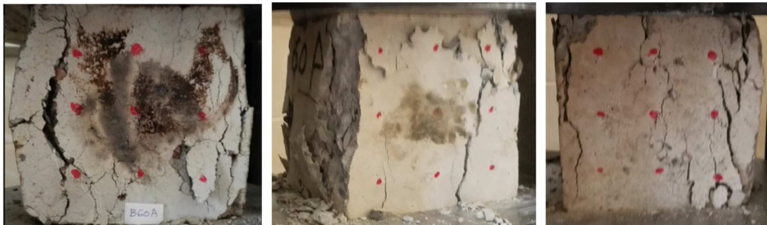
Figure 10 Concrete cubes after testing
